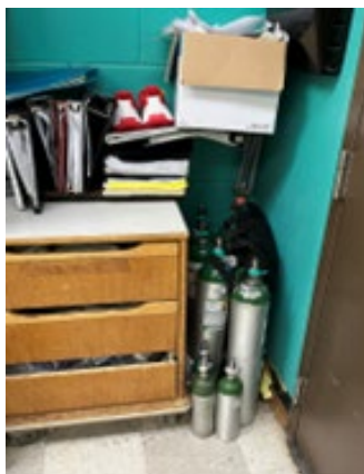
Photograph 7: Empty oxygen cylinders stored with full cylinders and missing signage.
