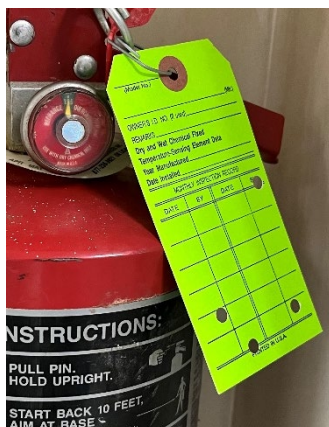
Photograph 5 (left): Fire extinguisher not inspected monthly.
