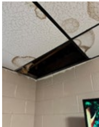
Photograph 1 (left): Missing ceiling tile.
